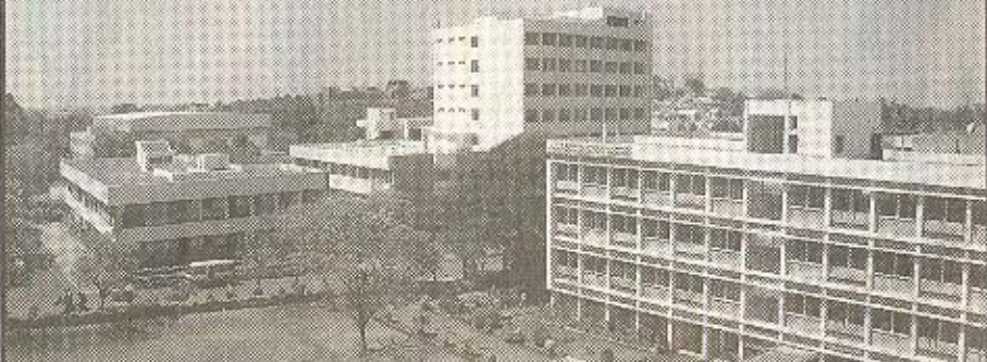
TOP VIEW OF B.M.S.ENGINEERING COLLEGE
